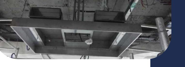
Operation ceiling is intended for supply of filtrated air into operating rooms.
